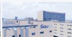
China Production Site
